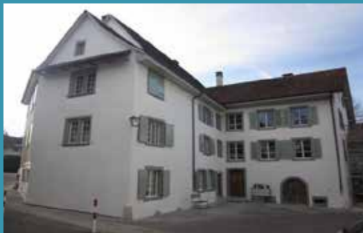
Fig. 3 The protected old mill in Sissach from the 13th century refurbished with aerogel render. Images: Kantonale Denkmalpflege Basel-Landschaft. [3]
