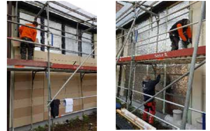
Fig. 1 exterior solution installation in Malmö (Sweden) demo site.
