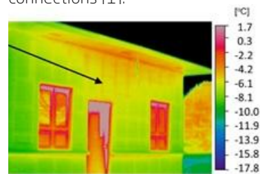
Fig. 1 Infrared imaging of a house insulated with VIPs. First wall retrofit with VIPs in the U.S.A.
