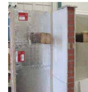
Fig. 1 The investigated T-shaped brick-wall with two wooden beams and two different VIP-systems as internal insulation separated by an internal wall
